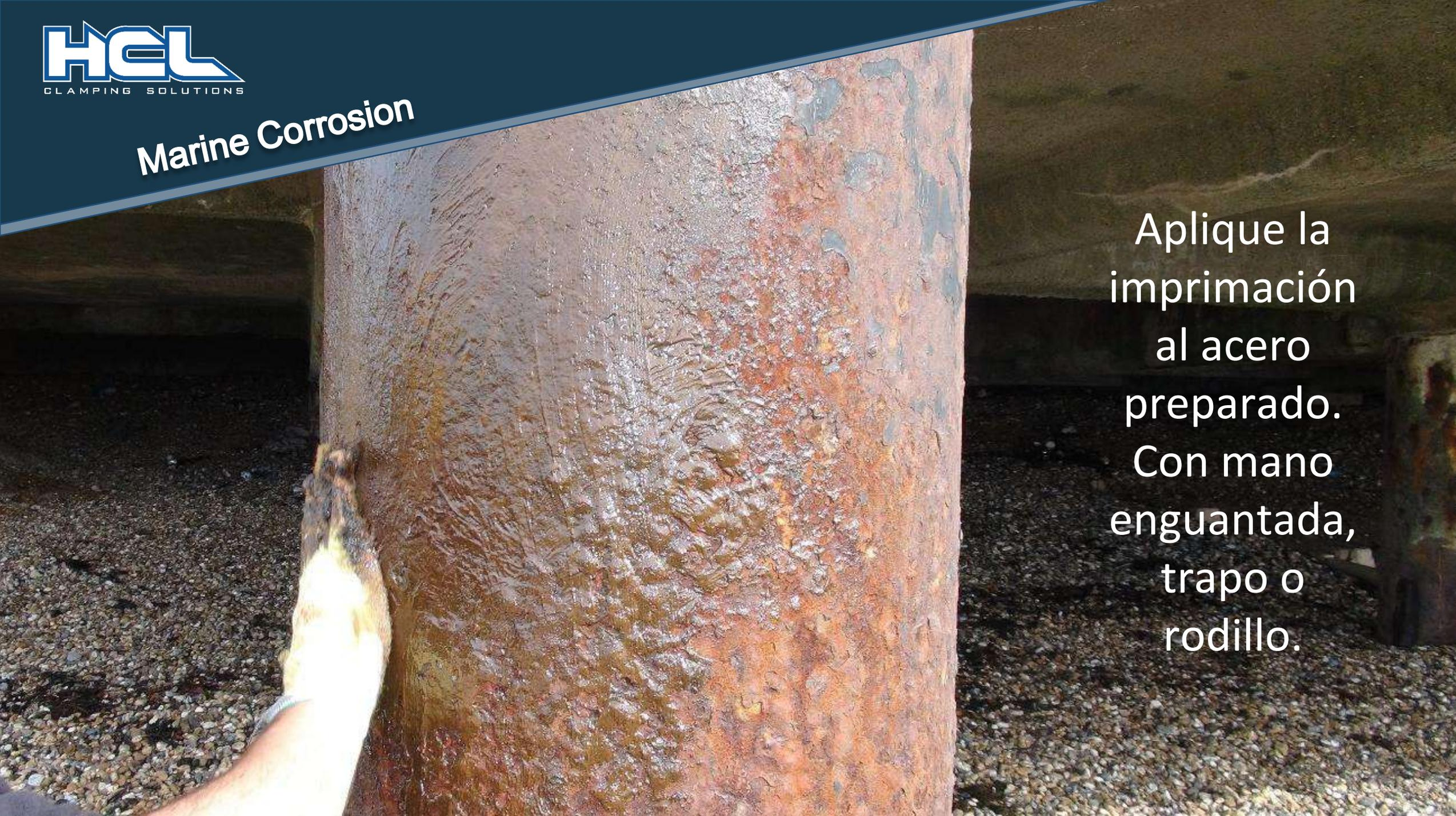
A close-up photograph showing a person's hand, wearing a yellow and white work glove, applying a greyish primer to a heavily rusted metal surface. The metal is a large, vertical cylindrical pipe or column. The background is dark and appears to be an industrial or construction site with gravel on the ground.
