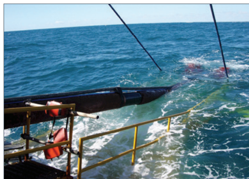
Smart® Band installed on Piggyback Pipelay operation
